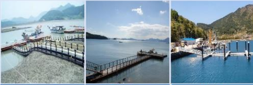
Berth facility Floating Mooring facility Yacht Mooring facilities
